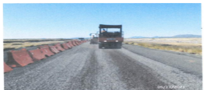
Figure 7. Application of the seal irrigation
