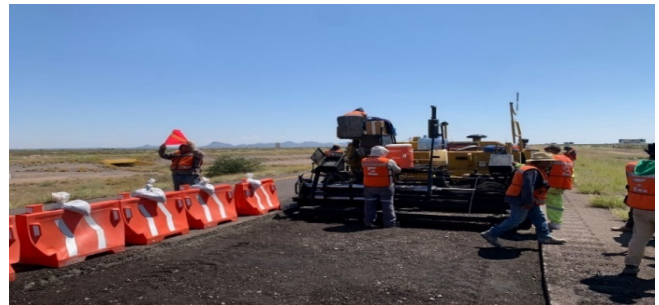
Figure 4 Foamed base paving with a paver
