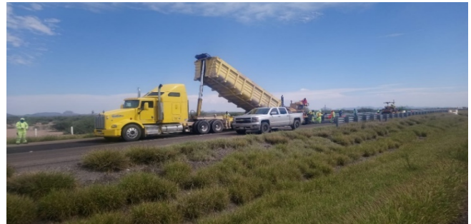
Figure 3. Truck emptying foamed base. The stabilized base is transferred to the site for paving with a paver
