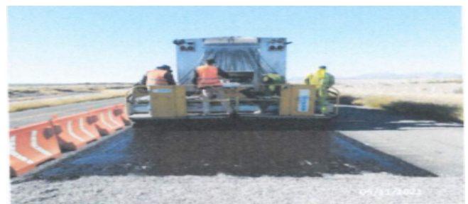
Figure 6. Application of seal irrigation
