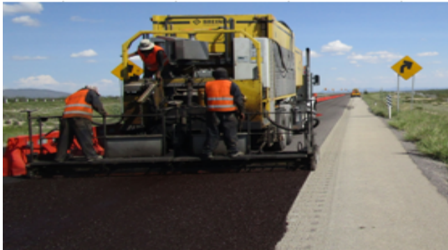
Figure 9. Application of the microagglomerate (During)
