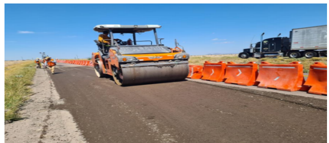
Figure 5. Compaction of the foamed base
