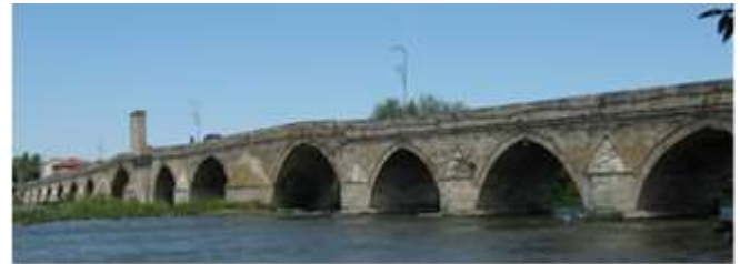
Figure 7: The Old Bridge.
