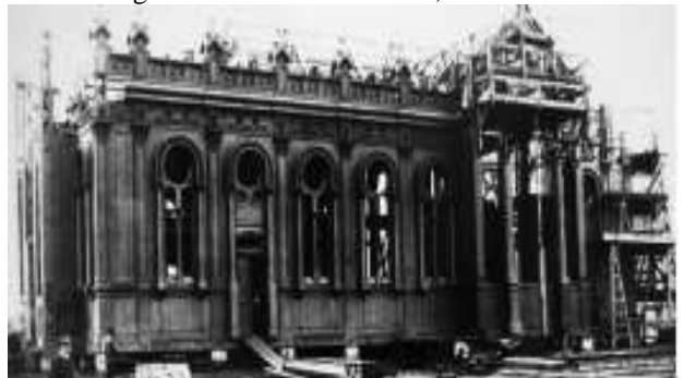
Figure 18: Construction phase of the church—iron structure
