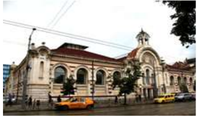
Figure 21: The front facade of the Central market hall
