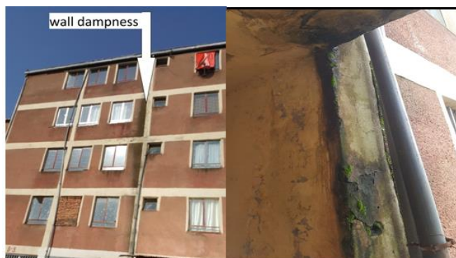
Fig 5. Wall dampness
