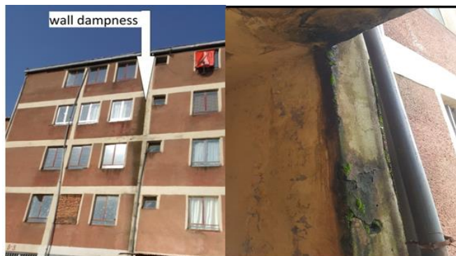
Fig 5. Wall dampness
