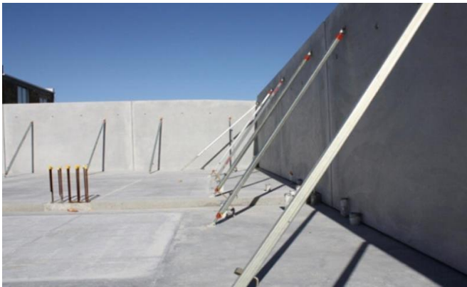
Fig 10: Fewer props required for precast concrete [3]
