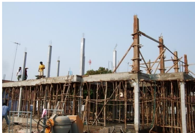
Fig 11: Shuttering and formwork in cast –in-situ [4]
