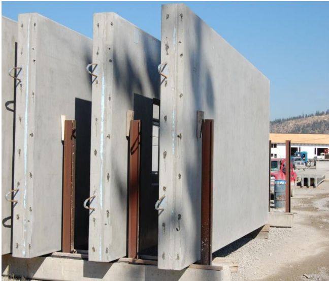
Fig 3: Precast Concrete Wall [12]
