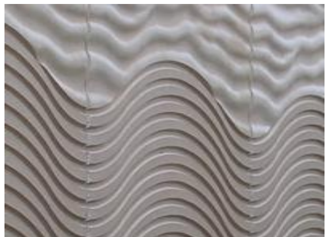
Fig 7: Precast concrete finished surface [2]
