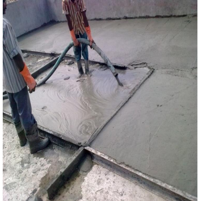
Fig 1: Cast-in-situ concreting method [5]
