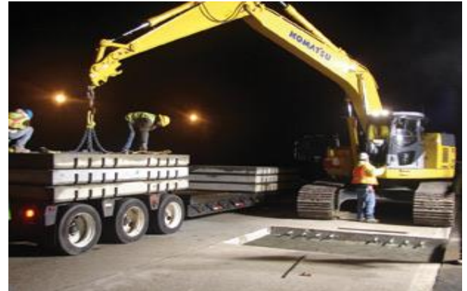
Fig 5: Lifting of precast members [9]
