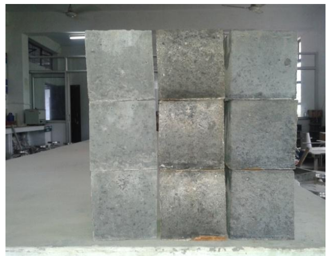
Fig. 5. Appearance of concrete cubes after withdrawal from 5%, 10% chloride solution and Tap water
