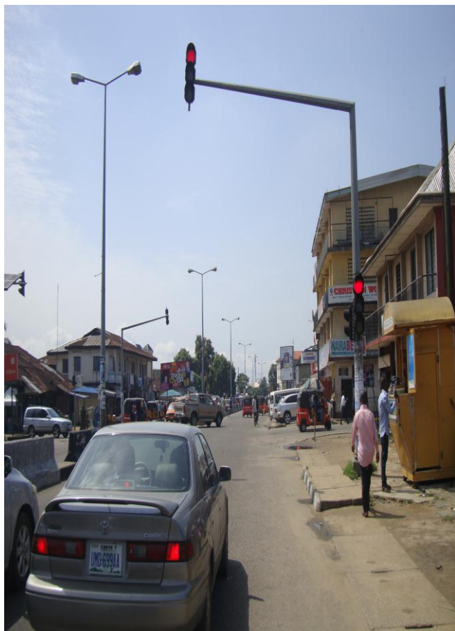
Fig. 2(a) Traffic Control point SP3
