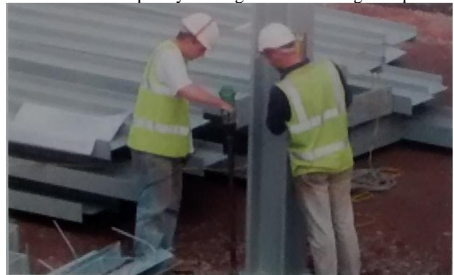
Fig.11: Tightening of anchor bolts
