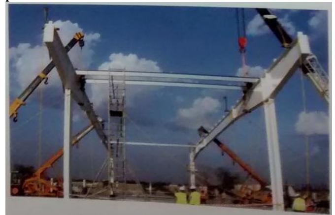
Fig. 6: Installing of 2 nd rafter
