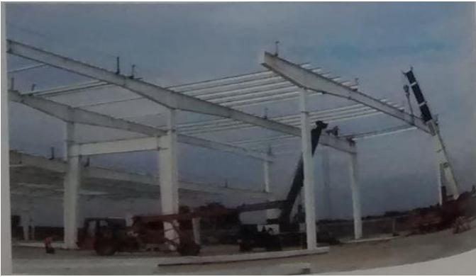
Fig. 7: Installation of bracing
