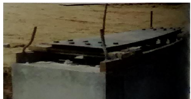
Fig. 2: Anchor Bolt Checking
