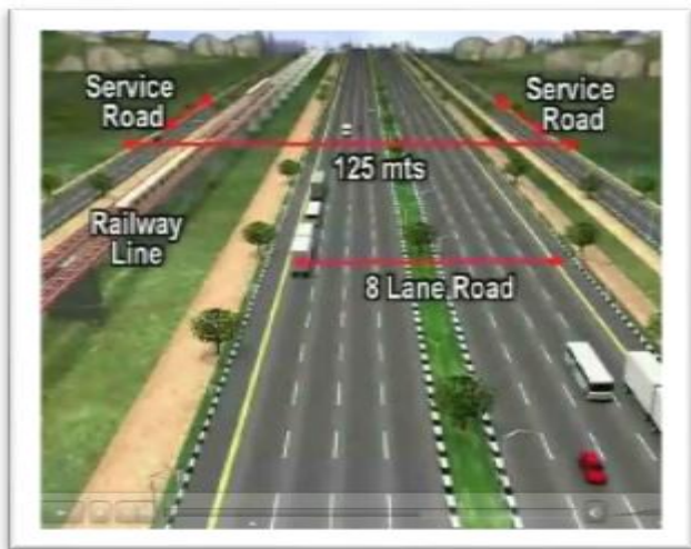
Fig 4.1 Outer Ring Road project of Hyderabad
