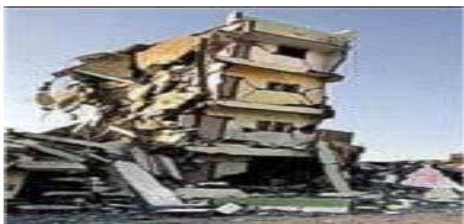
Fig.1 Failure of a residential building during the 2001 Bhuj earthquake (India)
