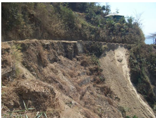
Plate 1. Retaining wall being constructed to check further subsidence along Lunglei road
