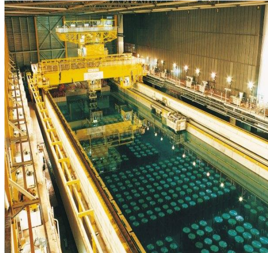
Fig: Storage pond for used fuel at the Thermal Oxide Reprocessing Plant at the UK's Sellafield site
