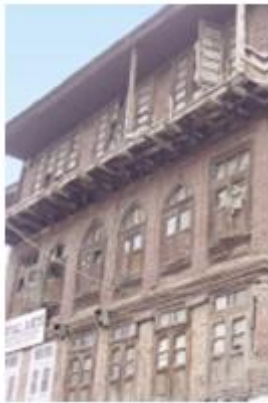
Fig. 2 Taaq type construction
