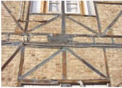
Fig. 1. Dhajji wall with baked bricks
