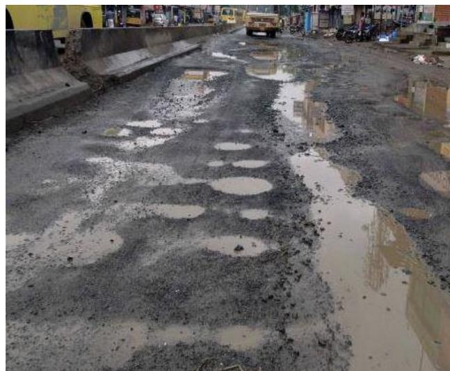
Figure II. Pits filled with water (damaged road)
